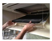
Filter Cleaning: Provided the grille catches are accessible, then open the grille/deflector assembly to the angle limited by the restraining straps. Remove and clean filter, replace making sure the grille catches are fully inserted into the fascia panel.
