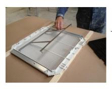
Commence by removing the return air grille (c/w with filter and security strap) from the cassette fascia panel
